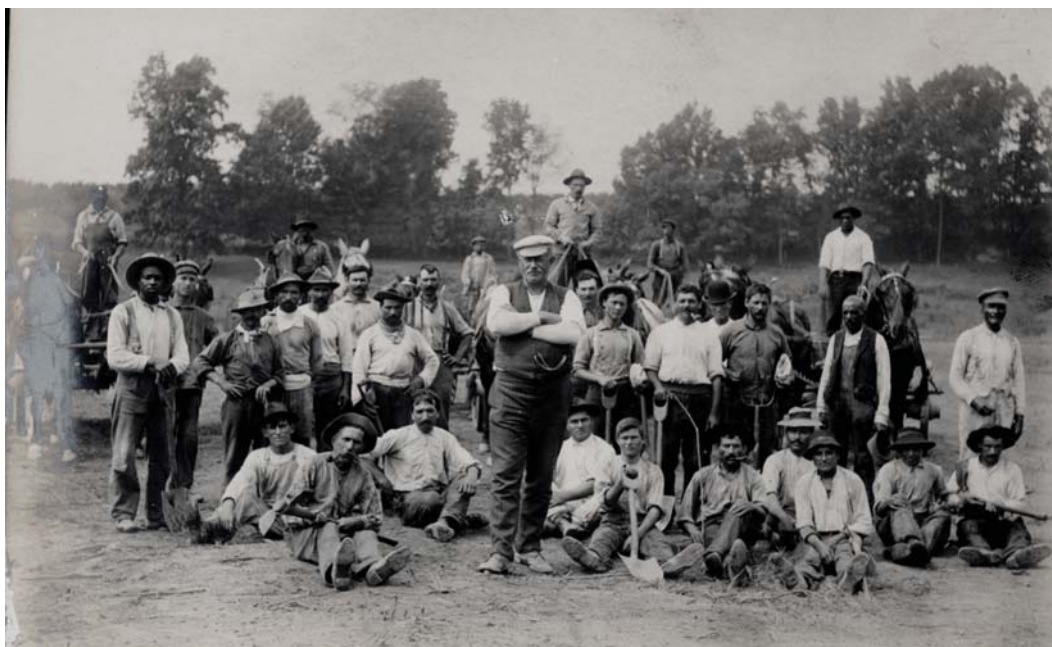
Item 46. Lake Carnegie construction workers.
